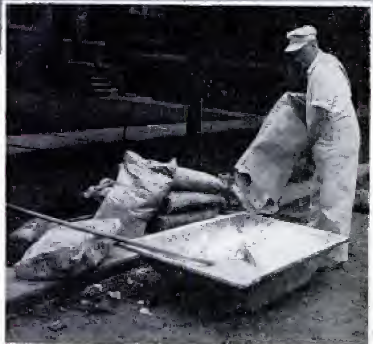
Base-coat plaster comes packaged with aggregate ready-mixed, requiring only addition of water. Reduces chances of error
